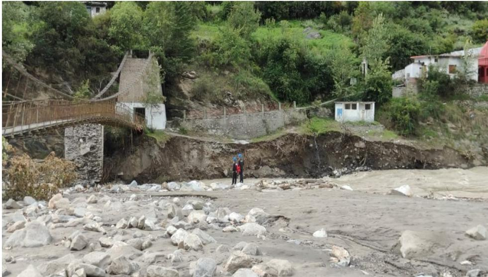
**Dharali debris flow can be termed as rainfall-cum-snowmelt water induced debris flow**
