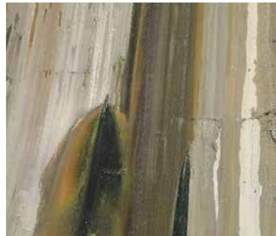
Fig. 2, 3 and 4 : Surface deficiencies on the downstream ogee of block 9.
