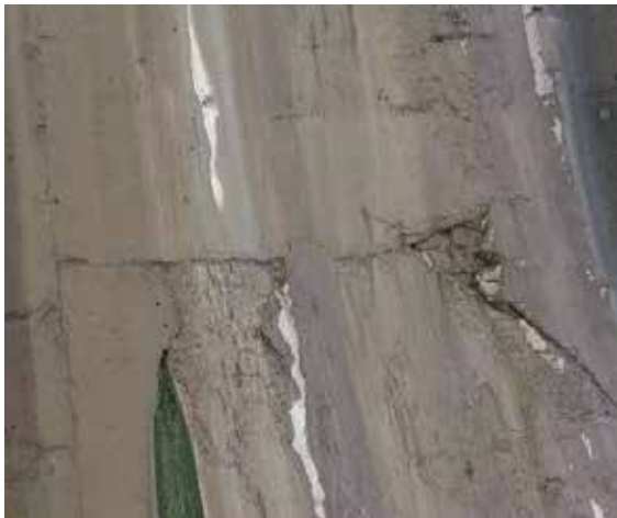
Fig. 2, 3 and 4 : Surface deficiencies on the downstream ogee of block 9.
