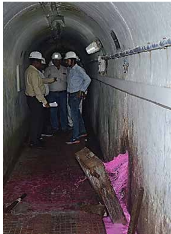
Fig. 1 : VPD at chainage 2136.6 m. in block number 9 showing flushing of water with dye
