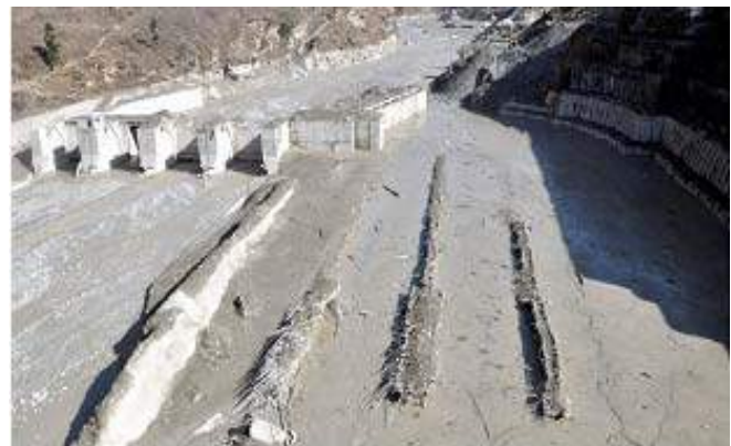
Fig. 4 : Washed away Tapovan Hydropower Project due to flash flood
