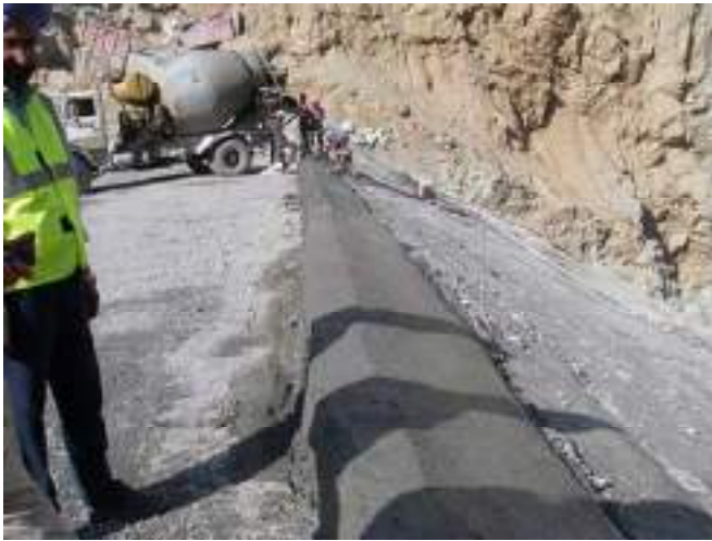
Figure 7 : Placement of Extruded Curb
