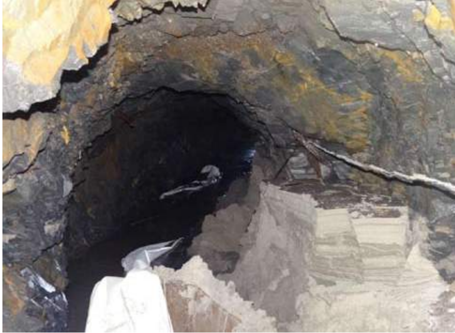
Fig. 7 : Silt deposited in exploratory drift of Power House during flood event of 2013
