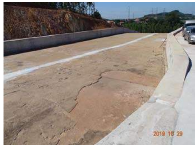
Fig. 7.2 : Khe Che Dam: the existing spillway has been widened (the white line shows the side wall of the original spillway)
