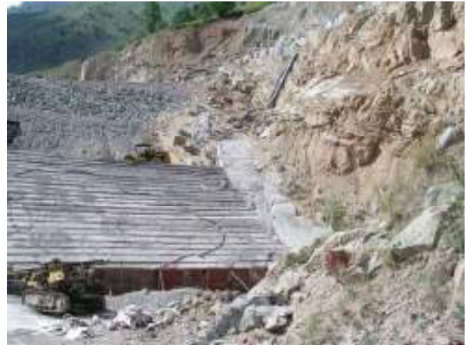
Figure 5 : Right abutment plinth
