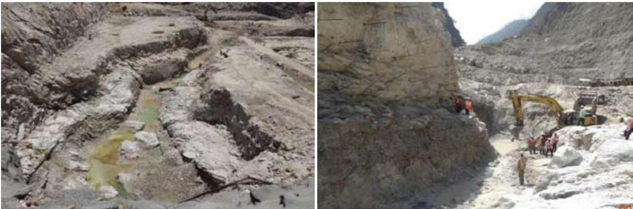
**Fig. 15 :** Shear zone trench excavation and rock anchor support on trench walls
