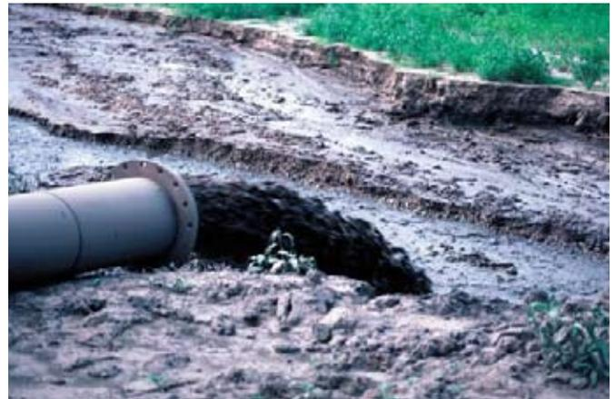
**Fig. 8 :** Illustration of Hydraulic dredging
