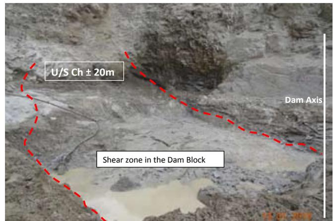
Fig. 12b : Close-up view of shear zone before final excavation and treatment
