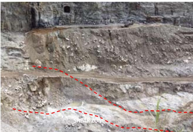
Fig.12a : View of shear zone before final excavation and treatment
