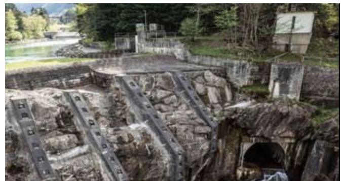
Fig. 4 : Sediment bypass tunnel operational since 1922 (pfaffersprung, switzerland. amsteg power plant)
