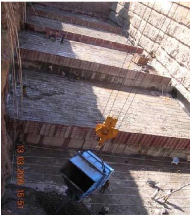
Fig. 9 : Photograph showing concrete placement and post cooling arrangement
