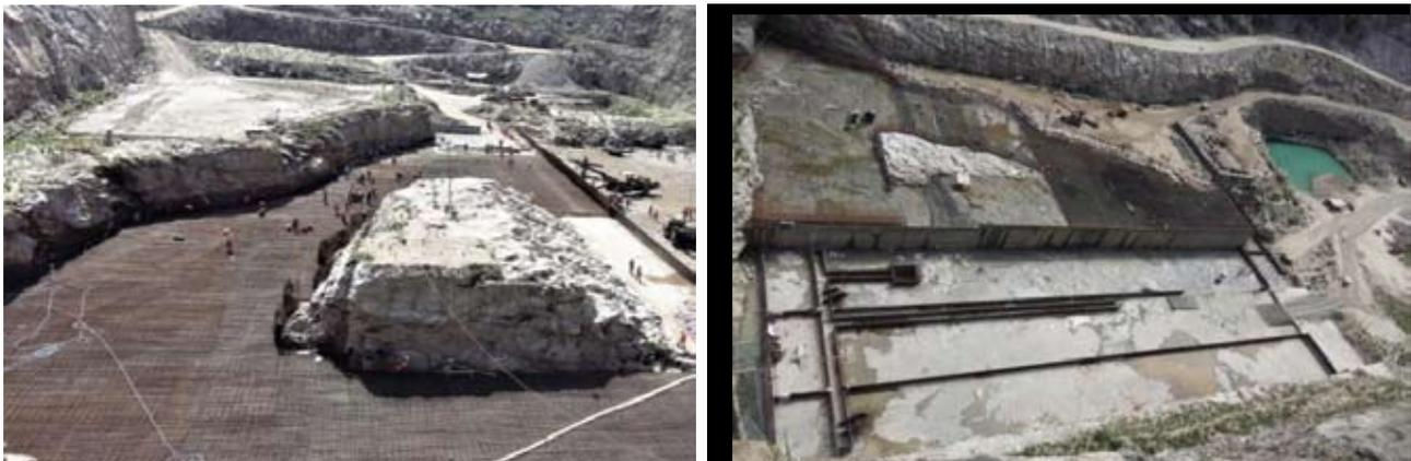
**Fig. 16 :** Treatment of shear zone at bottom (Left) and treatment at top (Right)
