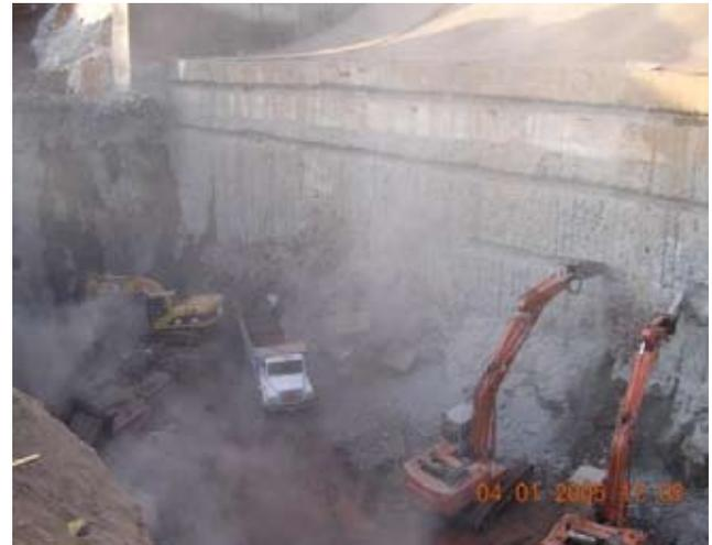
**Fig. 13 :** Cutting of Shear Keys
