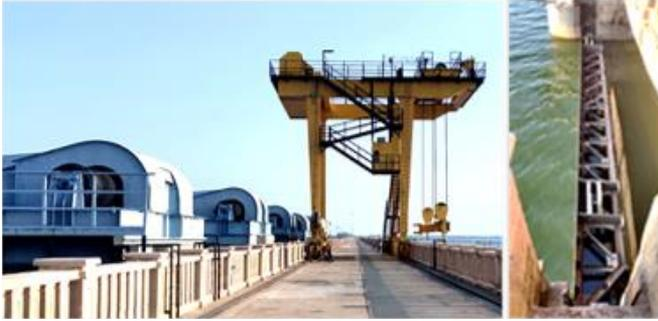
Fig. 8 : Narayanpur dam new gantry crane and set of stop logs
