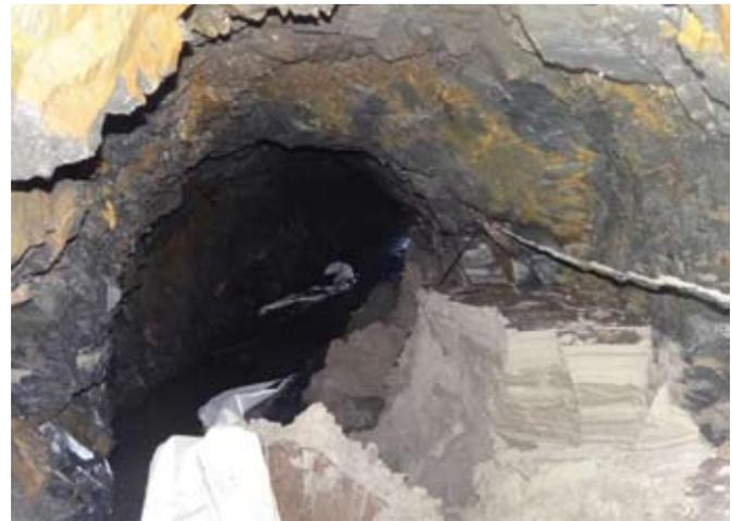
Figure 7 : Silt deposited in exploratory drift of Power House during flood event of 2013
