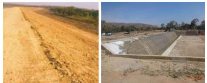
Fig. 7 : Sarathi dam raised and weir modified to ogee
