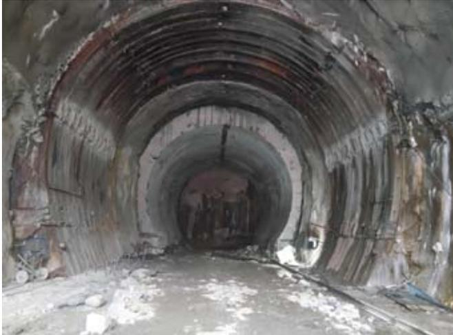
Fig. 6 : TBM Entry Adit with Launching Chamber
