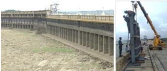
Fig. 9 : Replacement of 136 gates at KRS dam
