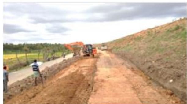
Fig. 12 : Mallaghata dam re-sectioning.
