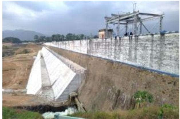
Fig. 11 : Pechiparai dam backing concrete.
