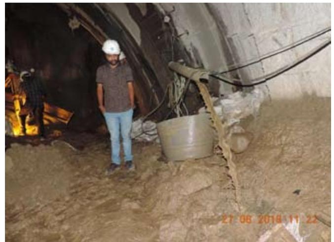
Fig. 5 : Gushing of water with silt from right side at RD 41.5m of TBM entry Adit
