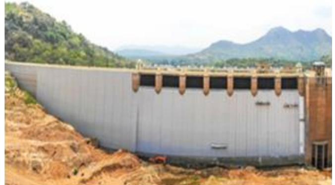
Fig. 15 : Servalar dam geomembrane treatment
