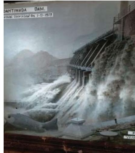
Fig. 7 : Dantiwada Dam – actual flood much more than the design flood
