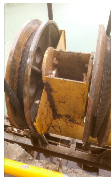
Damaged pulley cover
