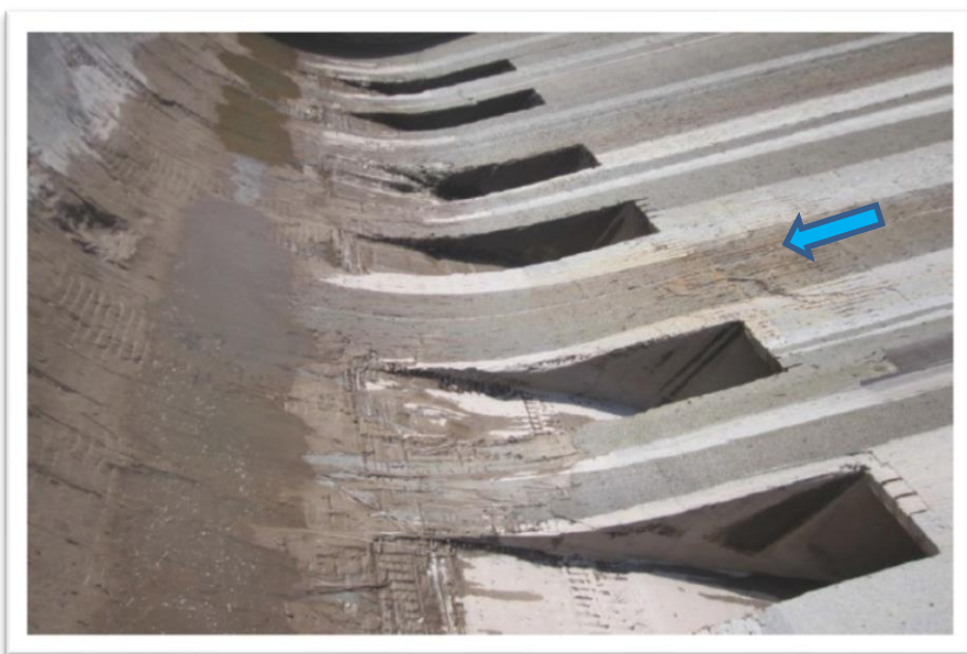
Erosion in the bucket area of Crest Spillway - Salal Dam
