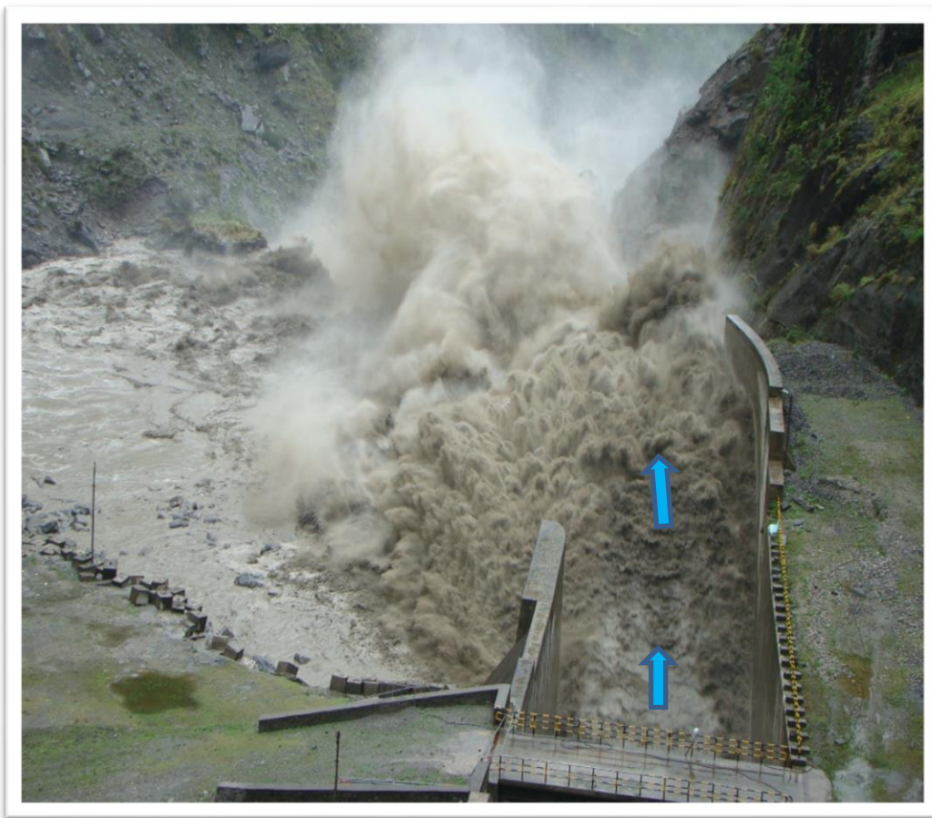
Spillway discharge: view from Dhauliganga Dam top
