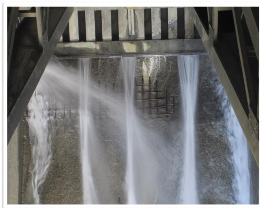
Water jet cutting near radial gate
