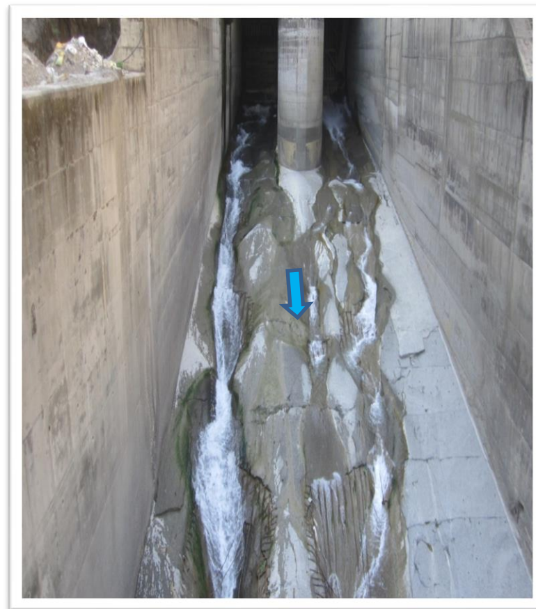
Damages on Spillway Glacis
