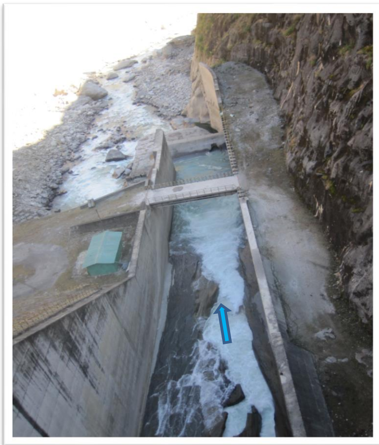
Damages on Spillway Glacis
