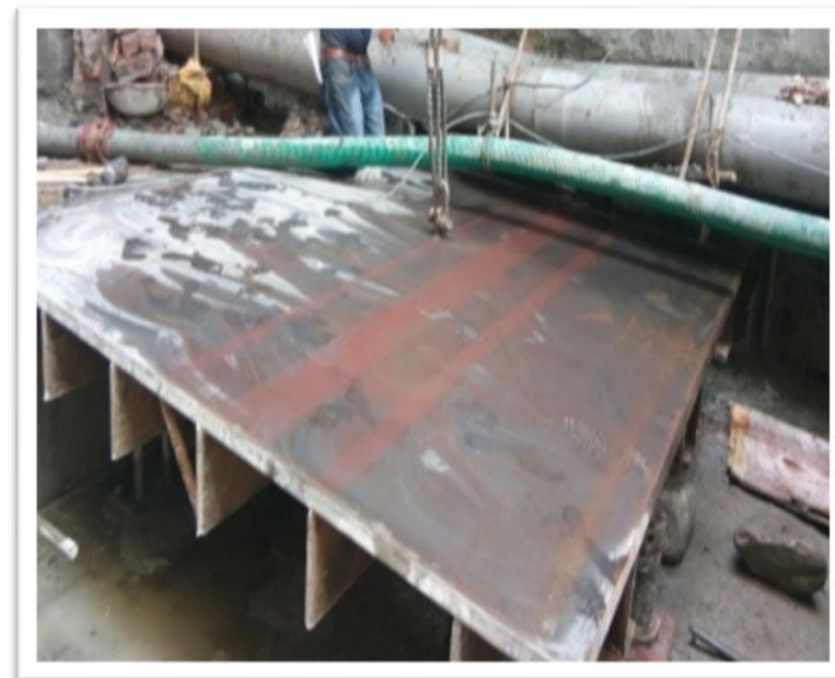
Stiffener under Steel liner
