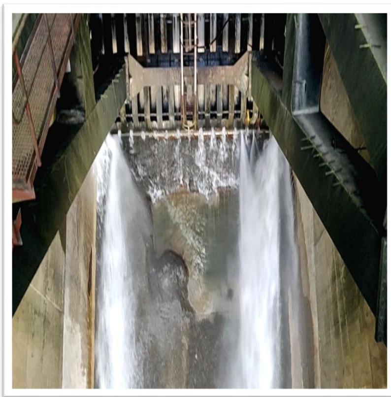
Damages on Spillway Glacis
