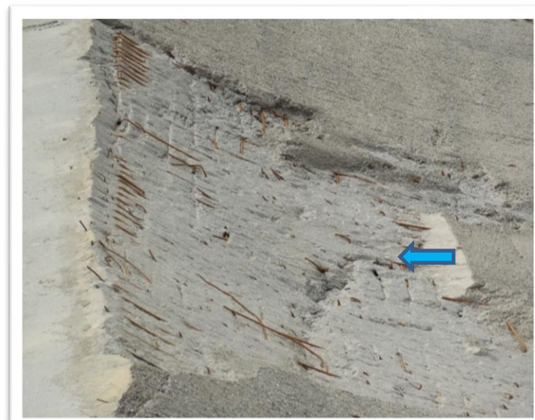
Erosion in the bucket area of Crest Spillway - Salal Dam
