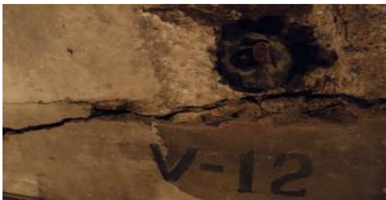
Down stream face of inspection gallery
