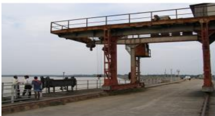
Top of Konar dam
