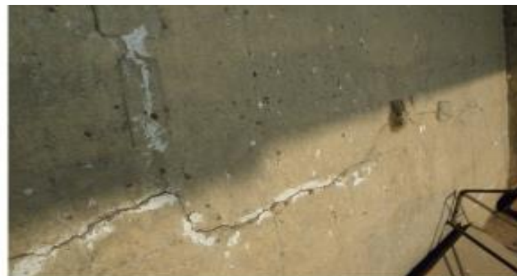
Outer dam body at abutment
