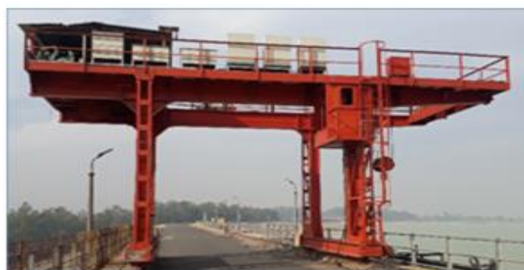
Renovated gantry crane
