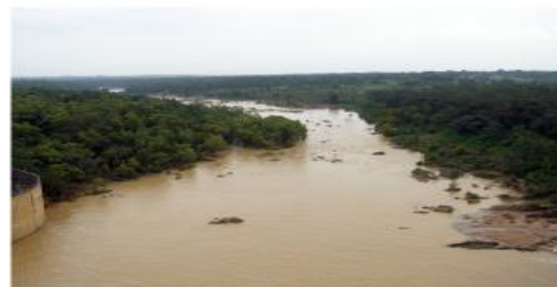
Down stream channel below Konar dam
