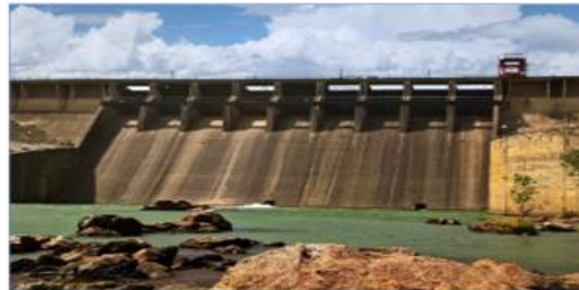
Leakage stopped in the control structure
