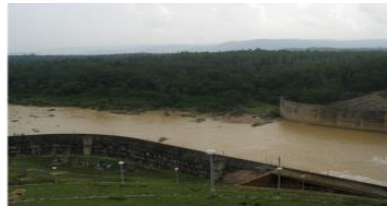
Down stream training wall of Konar dam
