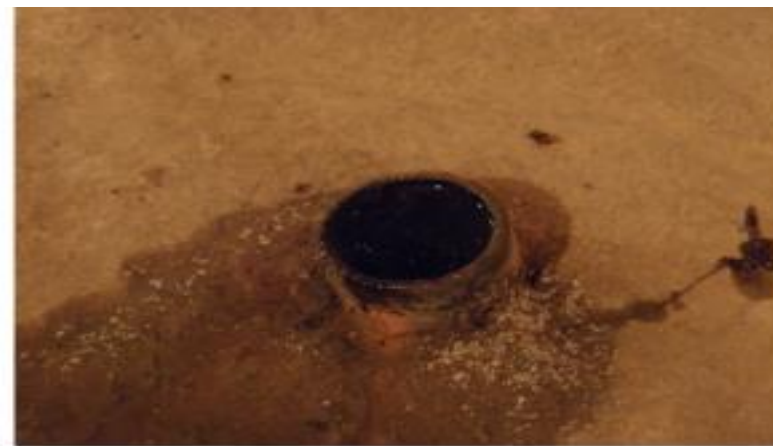
Drainage hole in drainage gallery
