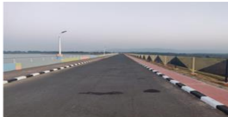
Repaired dam top road
