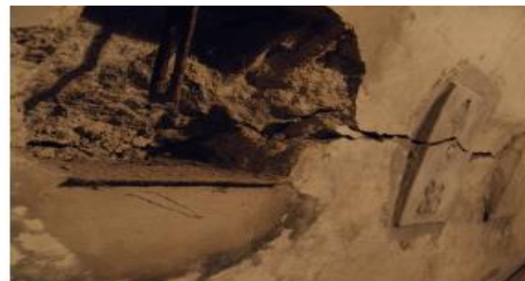
Down stream face of inspection gallery
