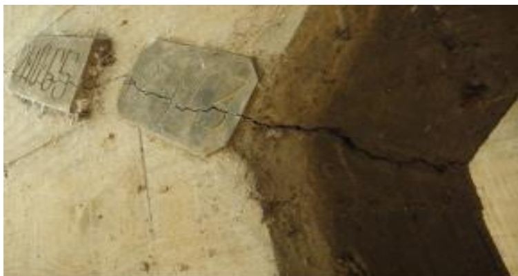
Outer dam body at abutment
