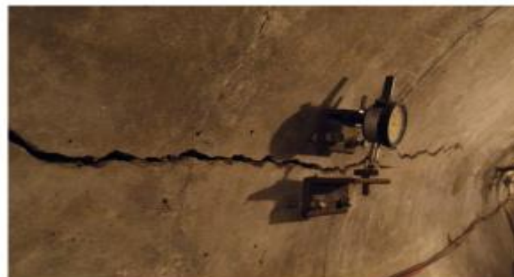
Down stream face of inspection gallery
