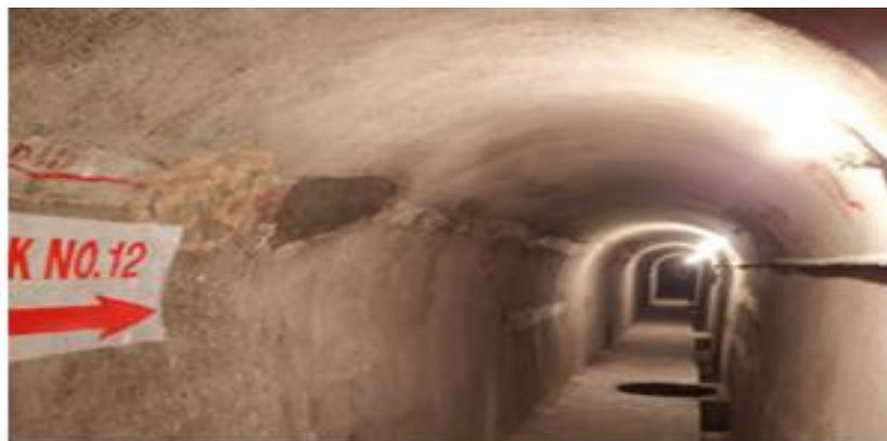
Gallery after grouting
