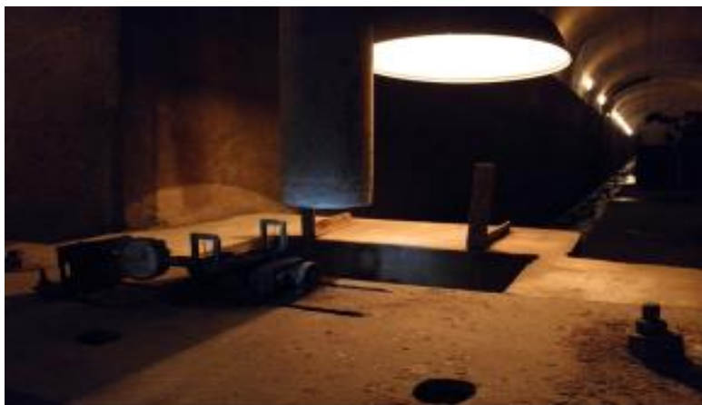
Plumb bob in drainage gallery
