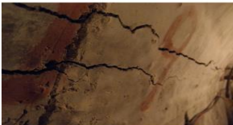
Down stream face of inspection gallery
