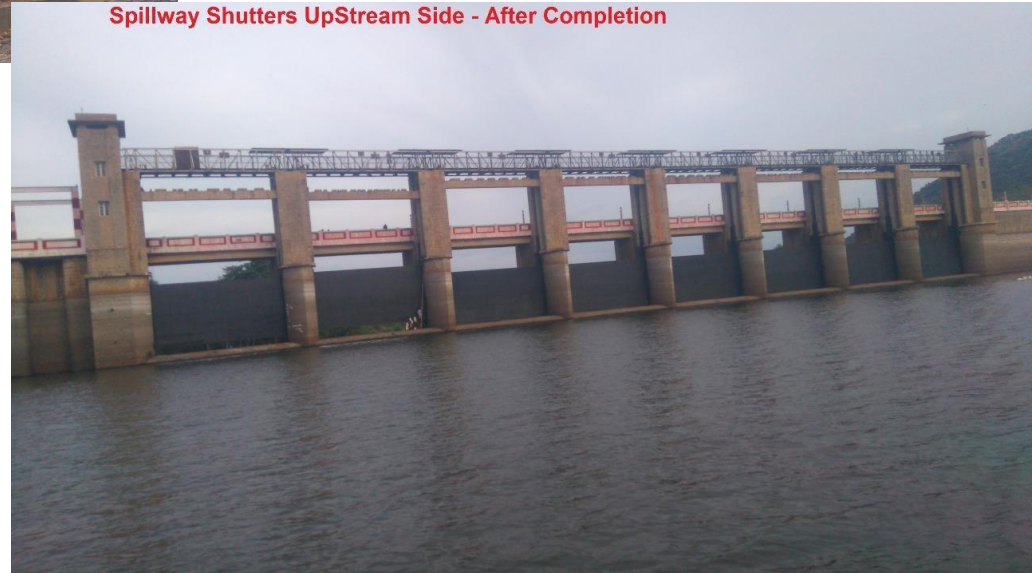
Spillway Shutters UpStream Side - After Completion
