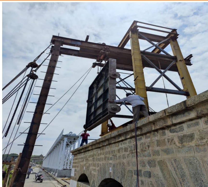
Removal of +114 Old Gate (from KRS Dam site erection)
