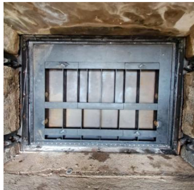
Leakage arrested +114' Level Gates after rehabilitation (from KRS Dam site erection)
