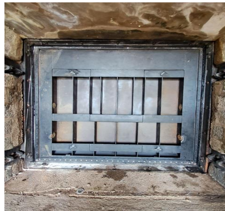
Erected of +114 New Gate (from KRS Dam site erection)
