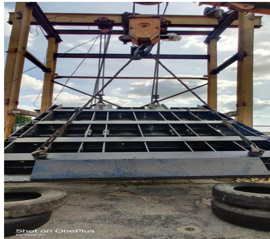
Erection of +106 New Gate (from KRS Dam site erection)
