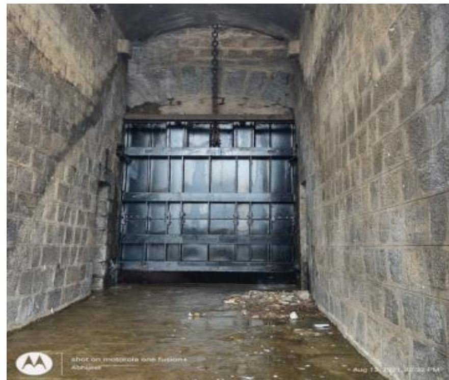
Leakage arrested +106' Level Gates after rehabilitation (from KRS Dam site erection)
