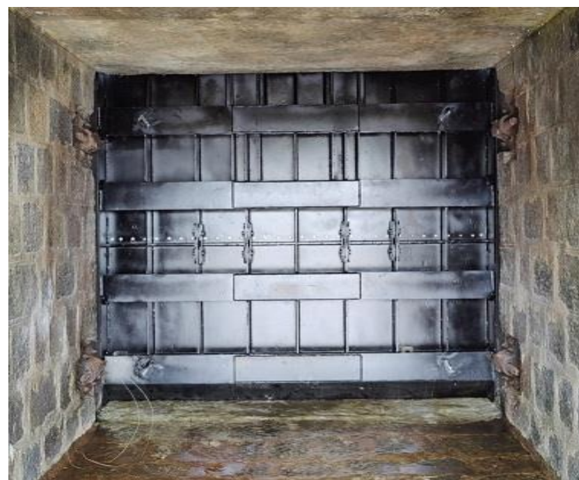
Leakage arrested +103' Level Gates after rehabilitation (from KRS Dam site erection)
