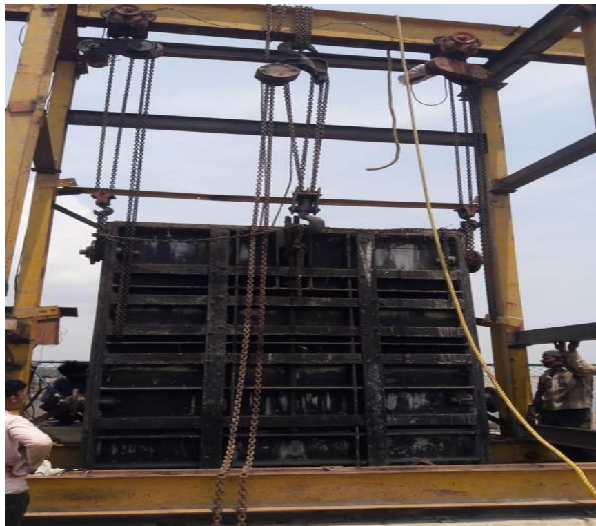
Removal of +106 Old Gate (from KRS Dam site erection)
