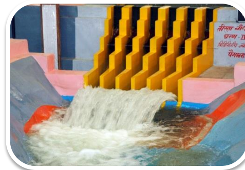
Reservoir & Appurtenant Structures
