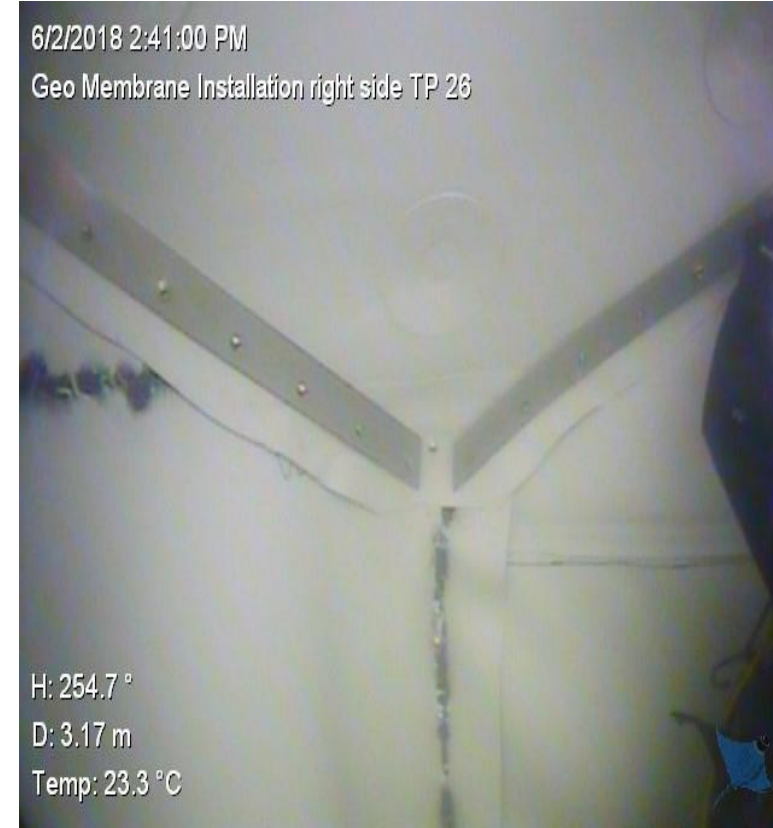
Installation of geomembrane
