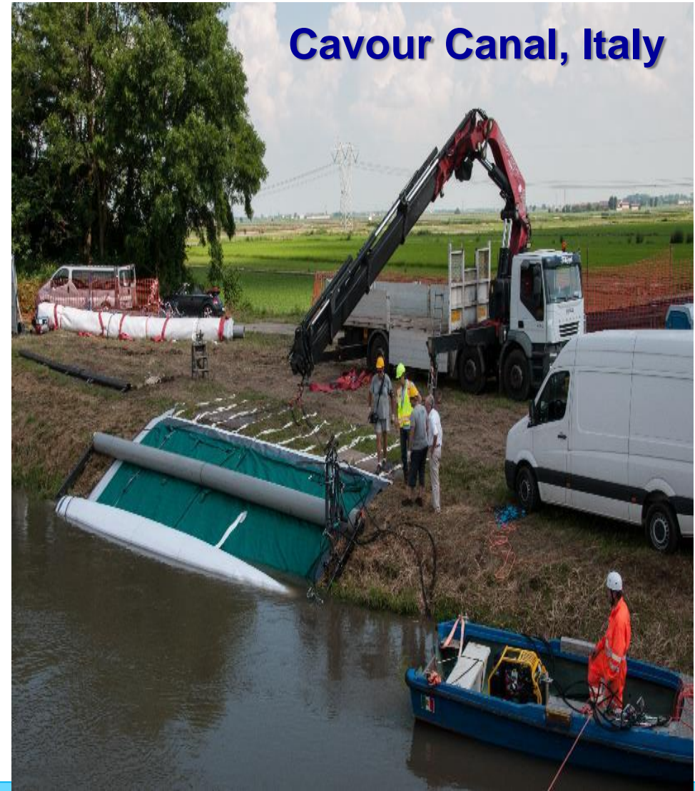
2 layers of geomembrane connected with strips
