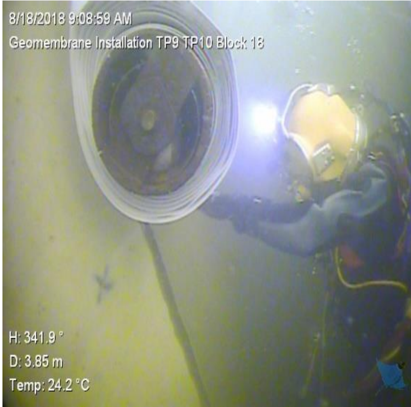
Installation of geomembrane
