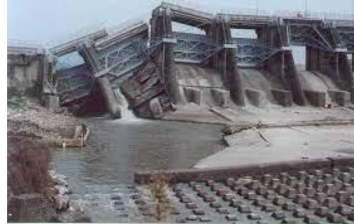
Shih-Kang Dam , Tiwan, Chi-Chi 7.7 MEQ, 2 bays damaged Bhuj, 2001, 7.7 M, dam in Kutchh, Crest settlement
