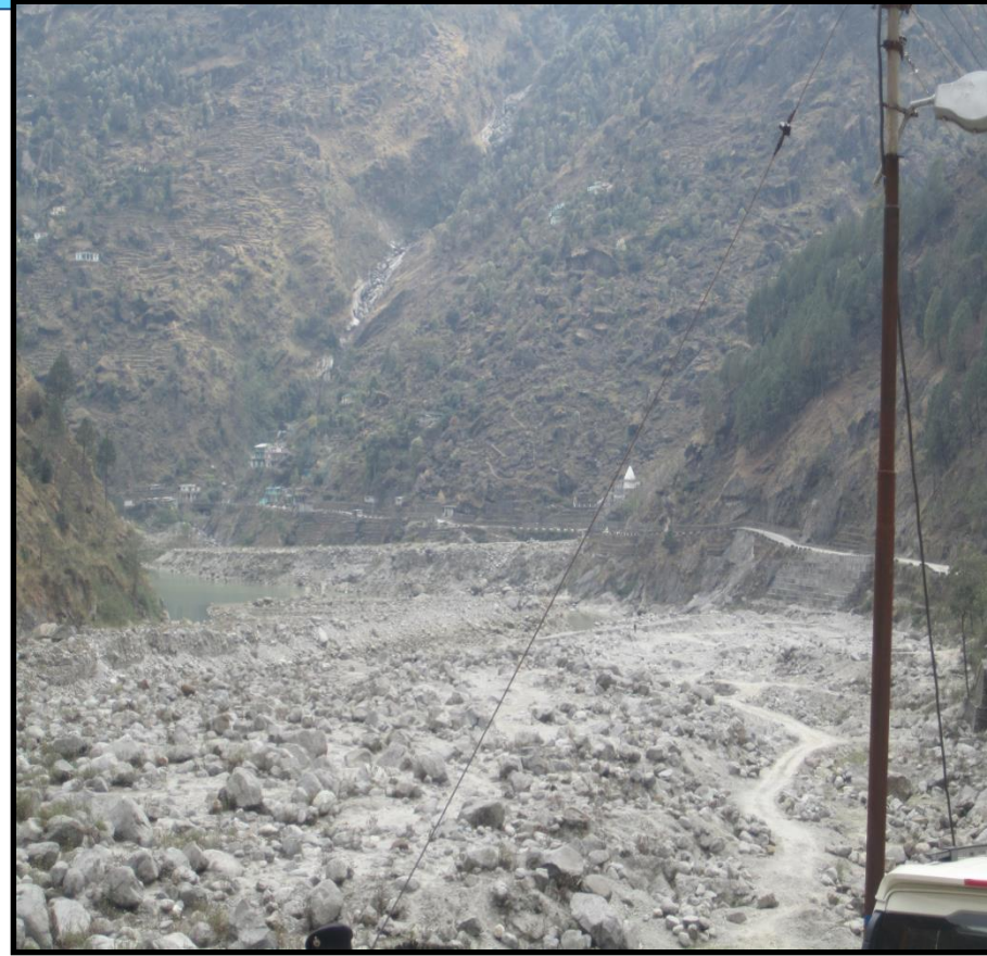
RBM filled at Reservoir Tail end
