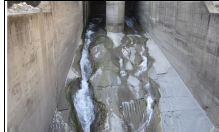
EROSION IN GLACIS OF DHAULIGANGA DAM SPILLWAY
