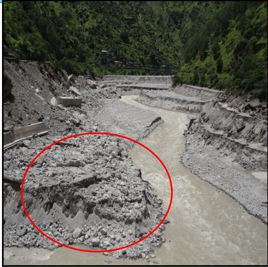
RBM filled in Reservoir Near Dam
