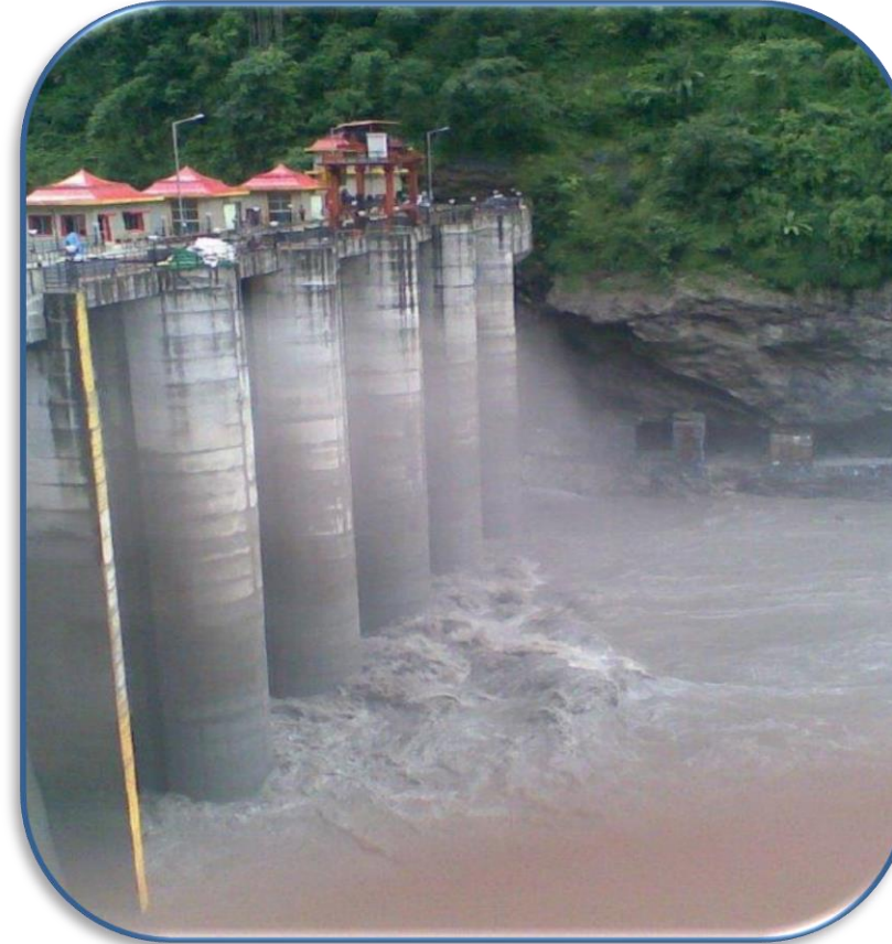
Huge Sediment deposition at Intake (2020-21)
