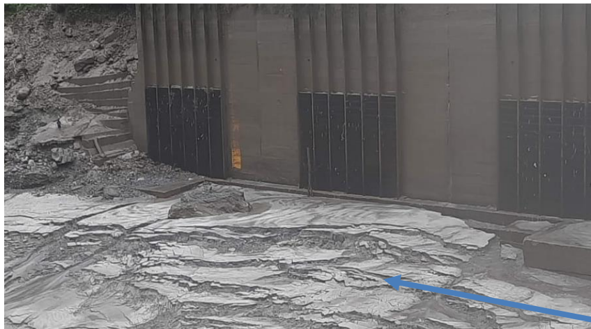
Huge Sediment deposition at Intake (2020-21)
