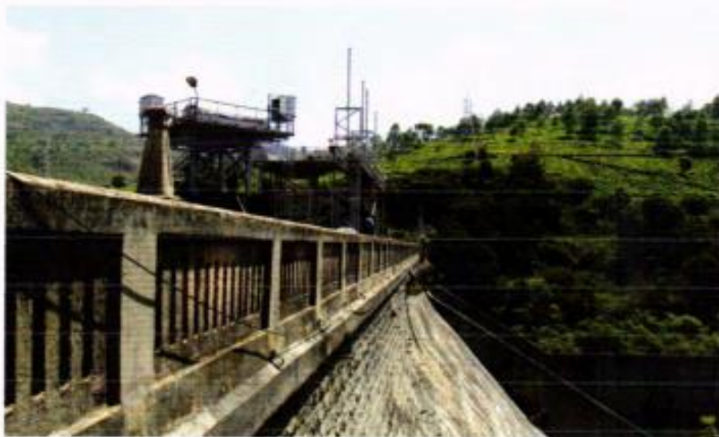
Kundah- Front view
