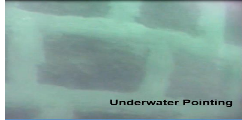
ROV for underwater racking & pointing work at Malaprabha dam, KaWRD
