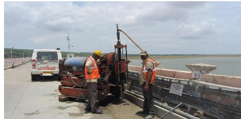
Dam body grouting with mix of cement, micro-silica (Almatti Dam, KaWRD).
