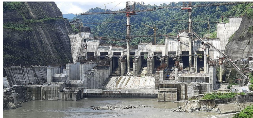
Side view of Dam showing additional base width
