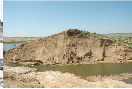
2010, Garada Dam 33m, Embankment
