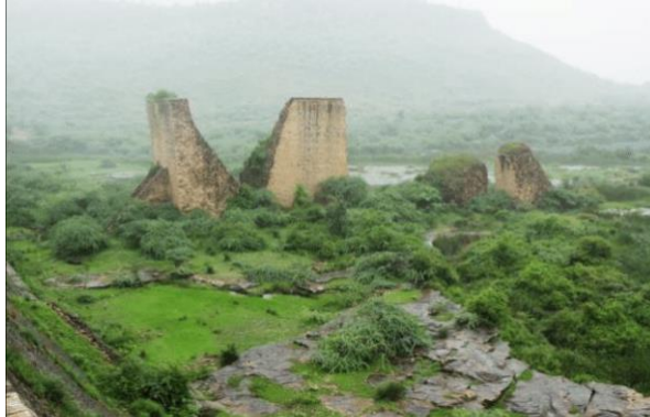
1917, Tigris dam 26m, Masonry
