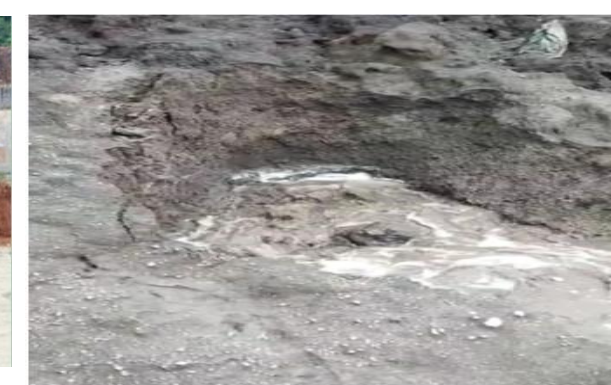
2022, Karam dam 52m, Embankment
