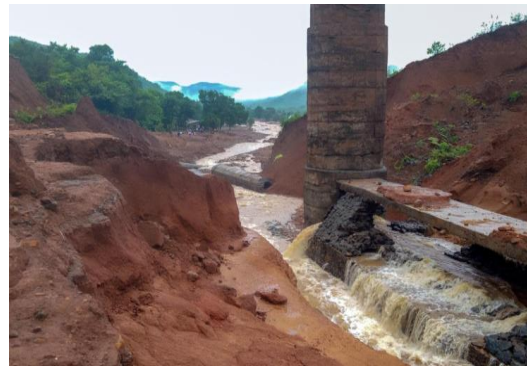
2019, Tivare dam 28m, Embankment
