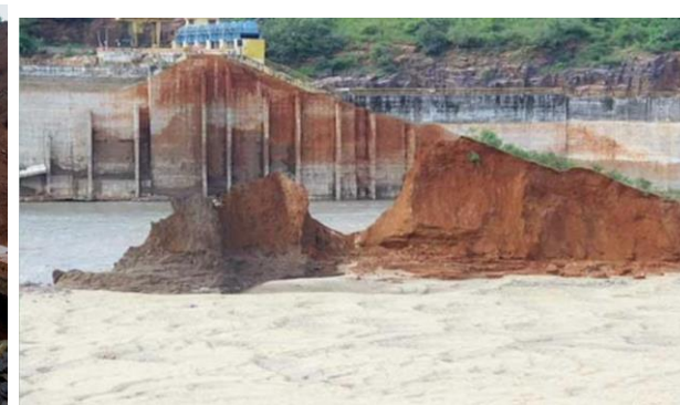
2021, Annamayya dam 25m, Embankment
