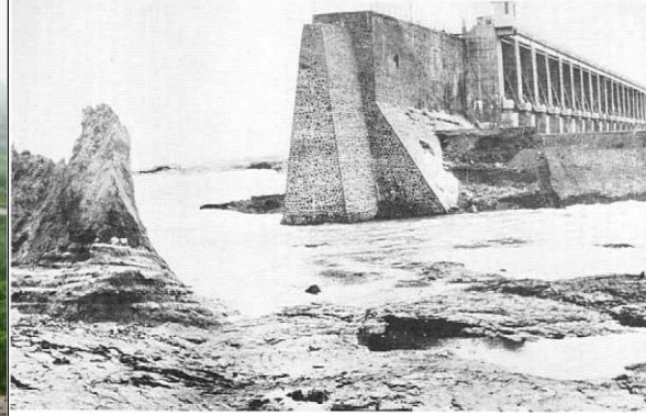
1979, Machhu II Dam 23m, Emb. Dam with Masonry Spillway
