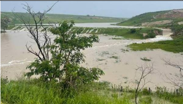
Igua dam – Brazil (December 2021)
