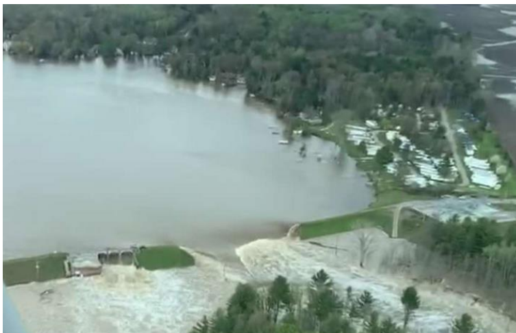
Edenville dam – USA (May 2020)
