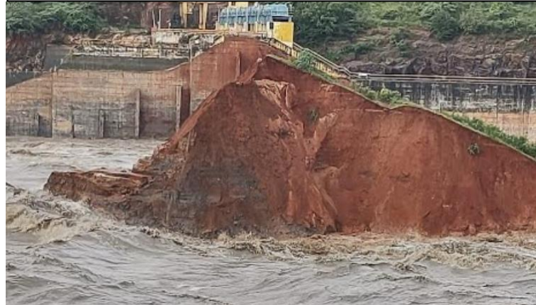
Annamayya dam – India (November 2021)
