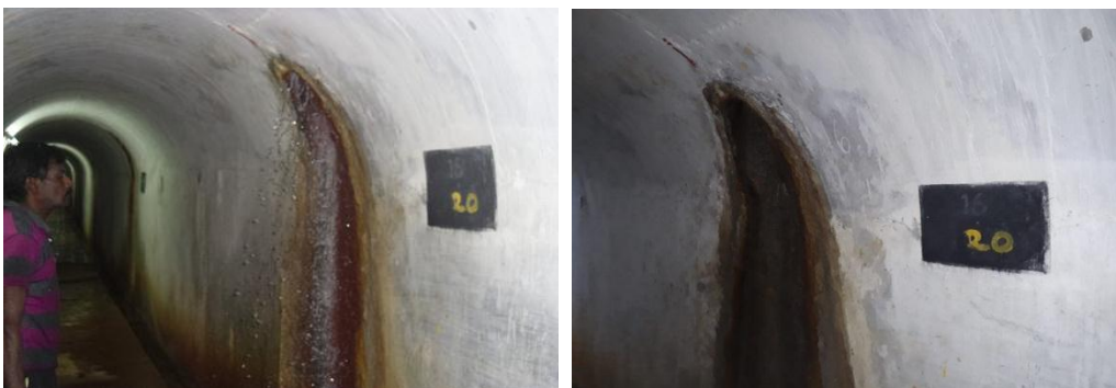
Figure 7. Vertical shaft leakage before and after geomembrane installation.
