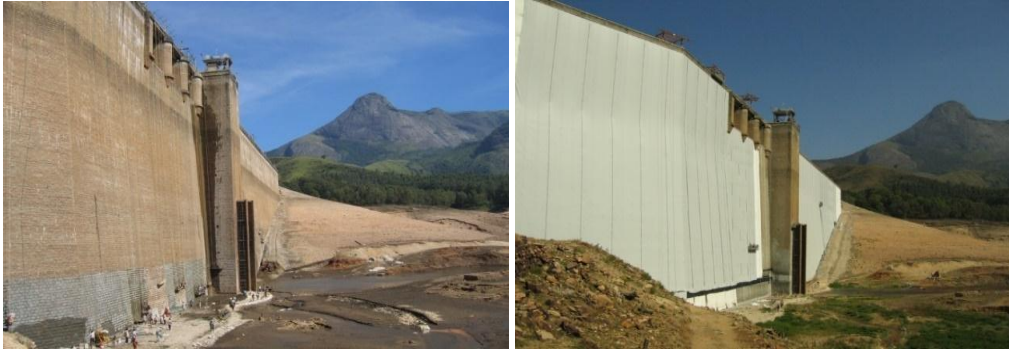
Figure 2. Upstream face of the dam before and after geomembrane installation.
