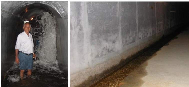
Figure 3. Drainage gallery before and after geomembrane installation.
