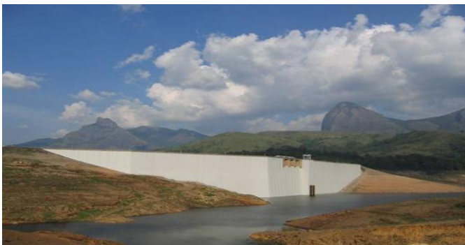
Figure 4. Kadamparai dam after installation of the geomembrane system.
