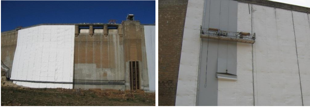
Figure 1. Installation of anti-puncture geotextile and of waterproofing geocomposite.
