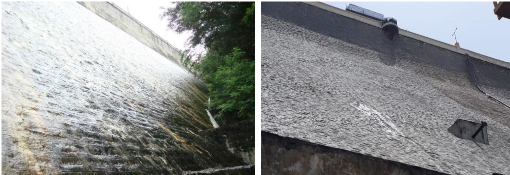
Figure 6. Downstream side before and after geomembrane installation.
