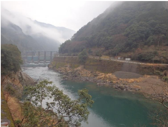
Figure 8. Sediment Replenishment at Downstream of the Setoishi Dam in 2018
