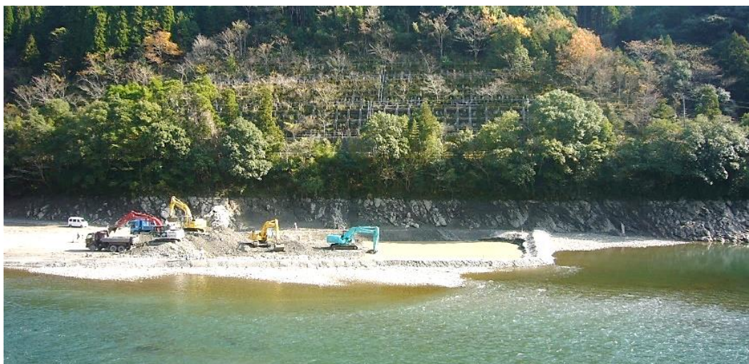
Figure 2. Excavation in the Setoishi Reservoir with emptying
