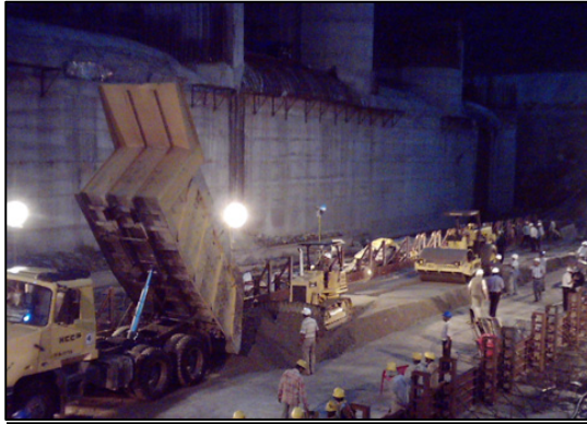
Photo 6 Concrete Placement
