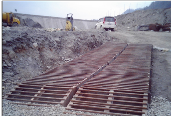
Photo 5 Washing Platform at RCC Pit
