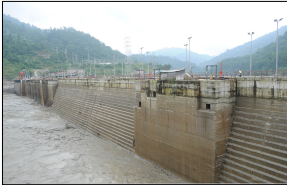
Photo 1 View of Upstream Face of RCC Dam and Entry of Fish Pass in
