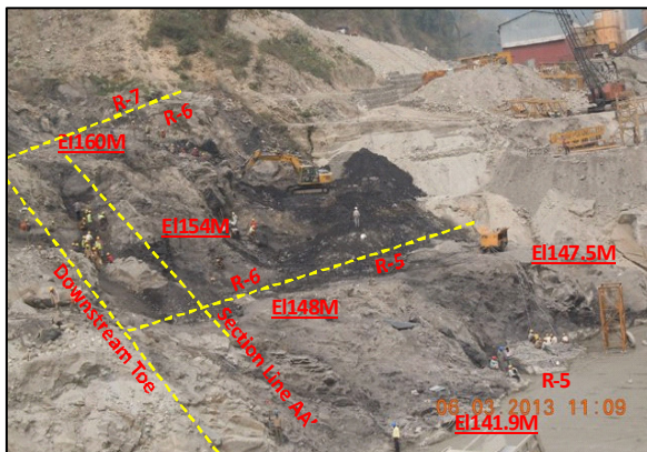
Photo 3 Foundation Preparation of RCC
