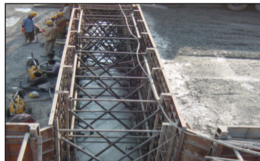
Photo 4 Gallery Arrangement Formwork and Precast Laying along with GEVR in Progress
