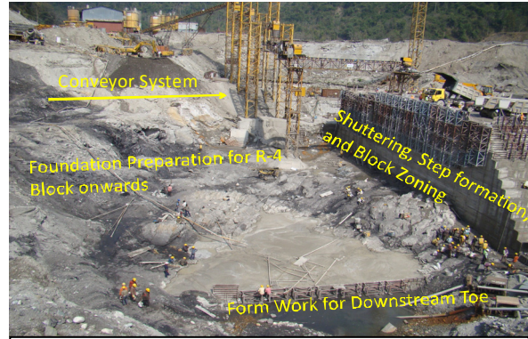
Photo 7 View of RCC Activities at Glance
