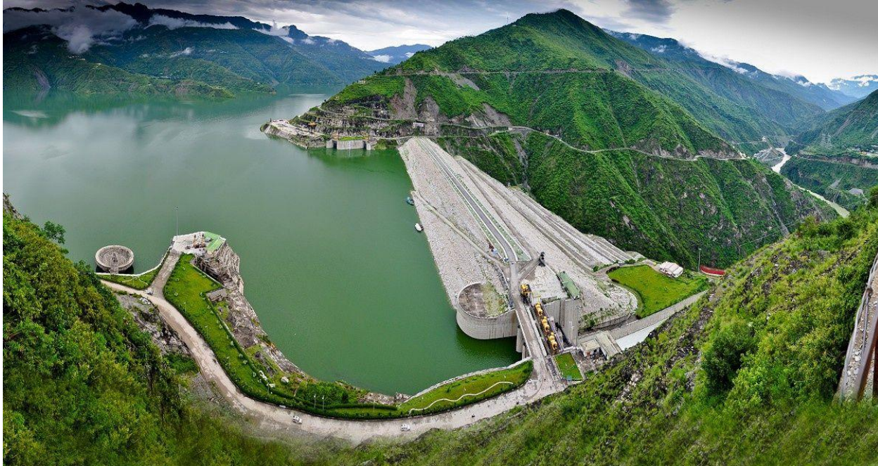
Fig. 2 : A View of Tehri Dam Project
