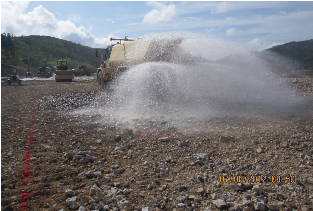
Photograph 2 : Water application on rockfill and compaction.
