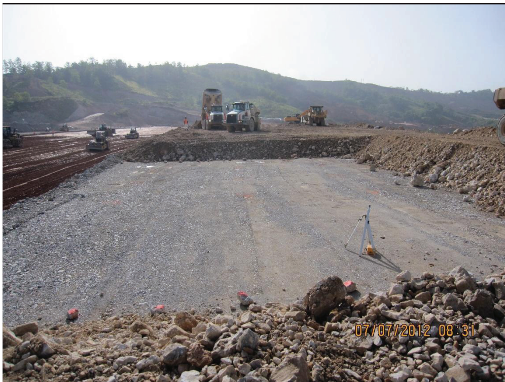
Photograph 1 : Test fill subgrade before rockfill placement.
