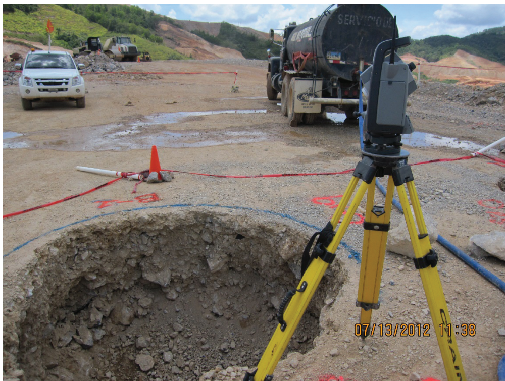
Photograph 5 : Excavation volume determination by scanning survey method.
