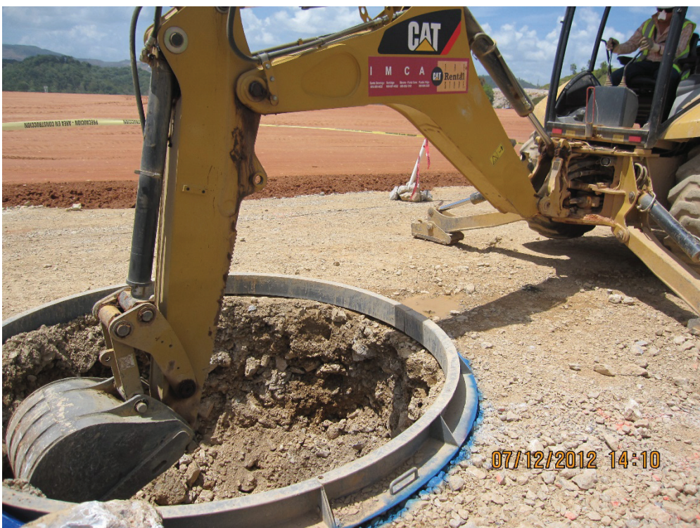
Photograph 3 : Backhoe excavation within steel ring for density tests.
