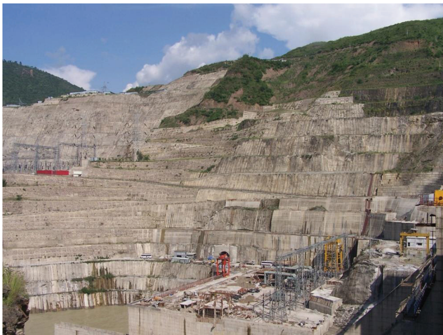
Figure 9 : Treated slope of right bank downstream of Dam axis
