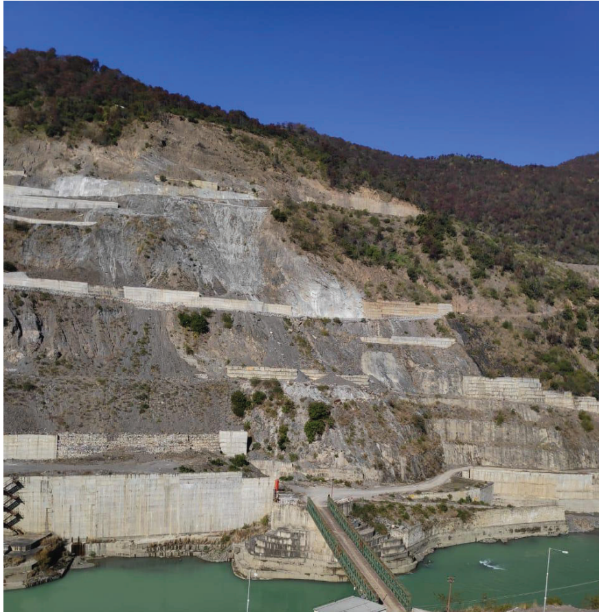
Figure 8 : Treated slope of left bank downstream of Dam axis
