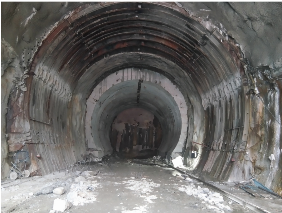
Figure 6 : TBM Entry Adit with Launching Chamber.
