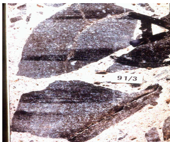
Figure 2 : Cracks in aggregates inside the concrete due to alkali aggregate reaction
