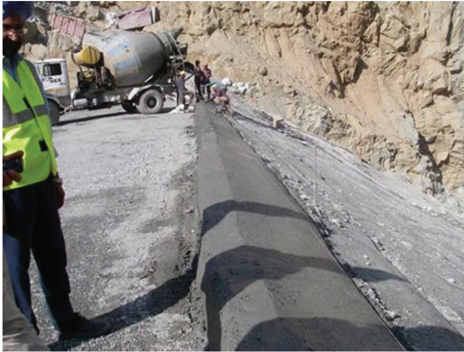
Figure 7 : Placement of Extruded Curb
