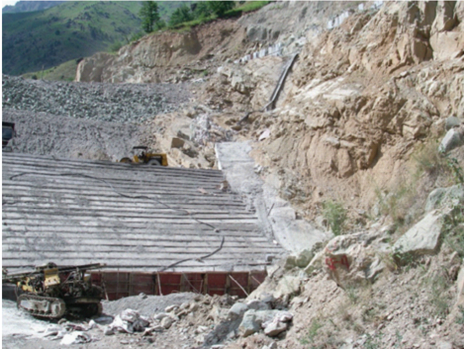
Figure 5 : Right abutment plinth
