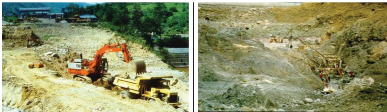
Fig 4 : Dam Excavation using CK-170 and 1025 tippers
