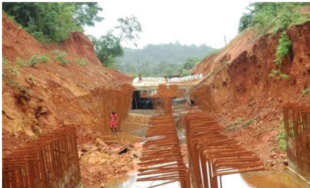
Photo 3 : The tilt and uplifting of the constructed culvert. Photo 4 : Benching of soil mass as a treatment to stabilizing the slope.
