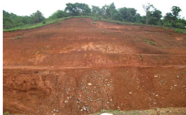
Photo 3 : The tilt and uplifting of the constructed culvert. Photo 4 : Benching of soil mass as a treatment to stabilizing the slope.
