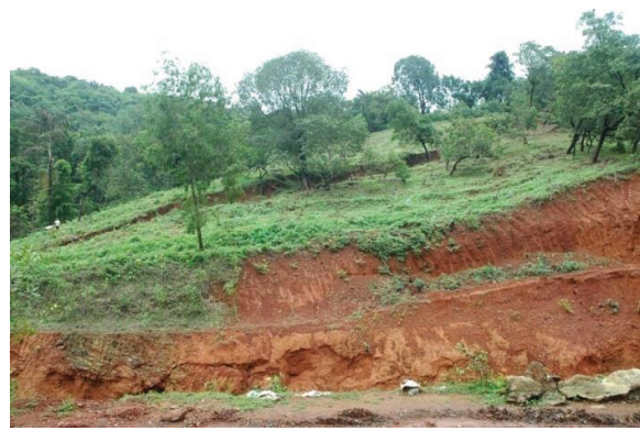
Photo 1 & 2 : Downward slide of overburden soil mass from tension crack.
