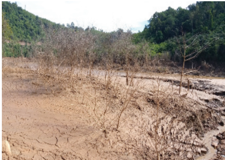
Figure 10 : Sedimentation in re-regulation dam reservoir in November 2017
