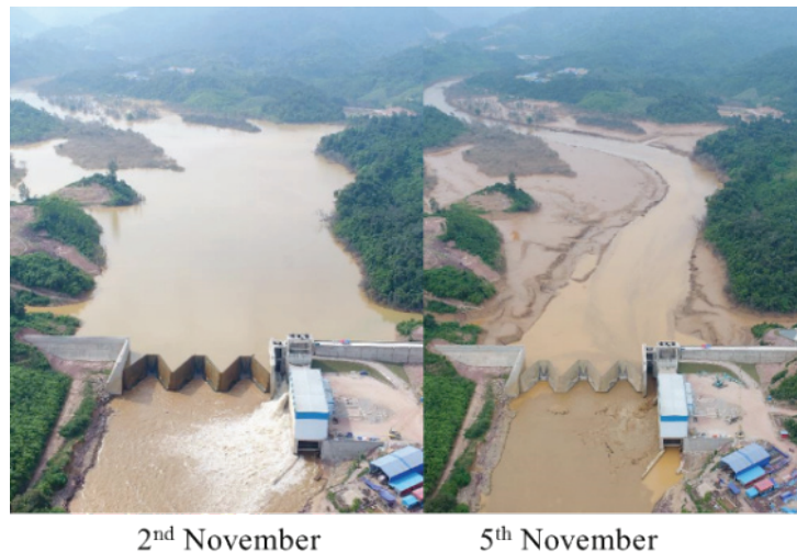
Figure 19. Photos of reservoir before and after sediment flushing
