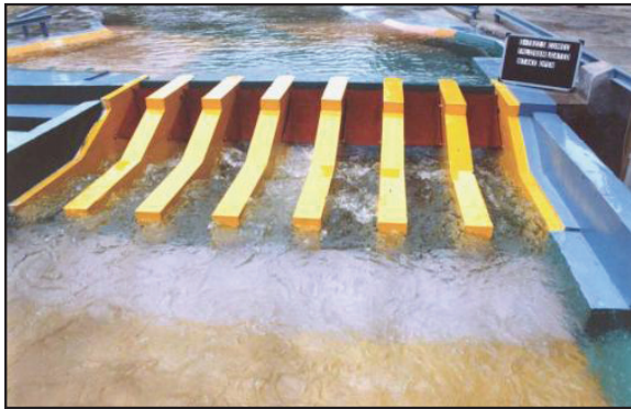
Photo 18 : Performance of stilling basin for the discharge of 7822.5 m 3 /s for gated operation of spillway
