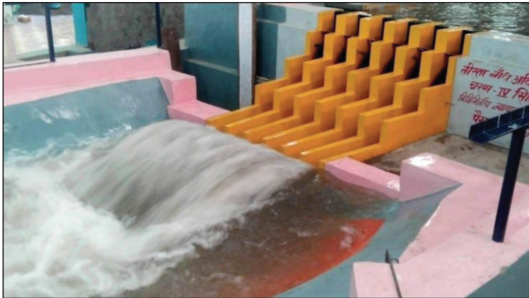
Photo 3 : Performance of energy dissipator for the discharge of 13000 \text{ m}^3/\text{s}
