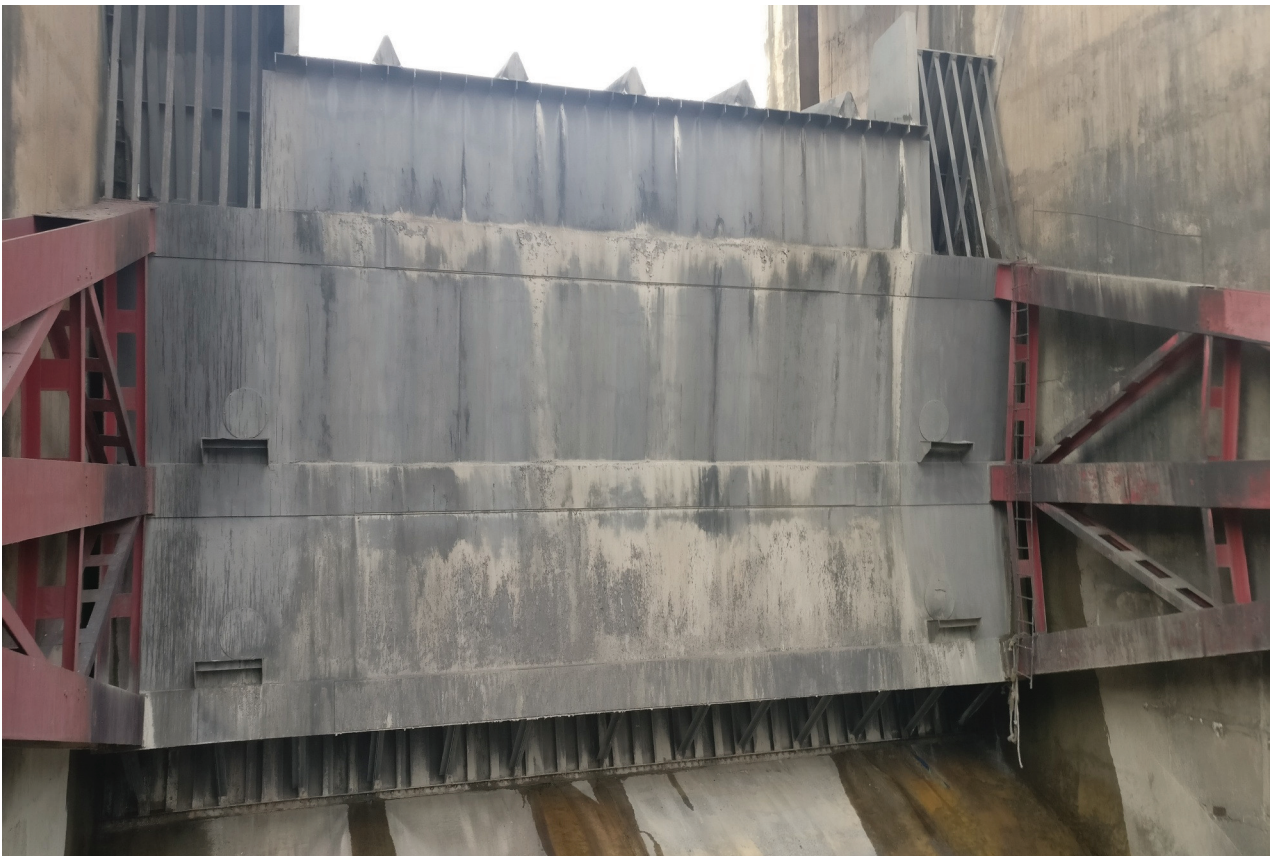
D/S VIEW OF OLD RADIAL GATE NO. 12
