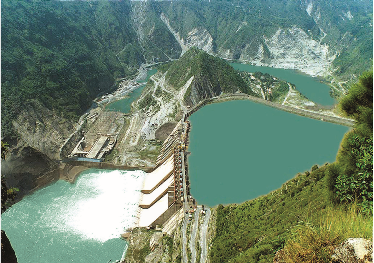
ARIAL VIEW OF SALAL PROJECT
