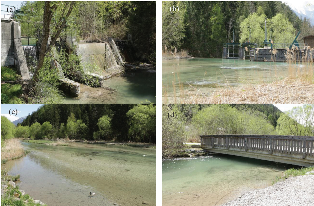
Figure 1 : (a) Gaulwerk weir with two gates and two overflow sections, (b) view downstream from reservoir to weir, (c) view upstream from weir to reservoir. Reservoir completely filled with sediments, d) Knappenwelt Bridge at the reservoir head with almost no freeboard left between bed and bridge. Photographs by C. Auel.
