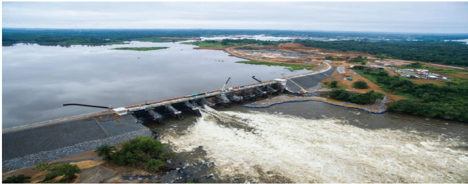
Figure 5 : MCHPP Spillway Flow of Water during the Raining Season (Source: LEC-PIU)
