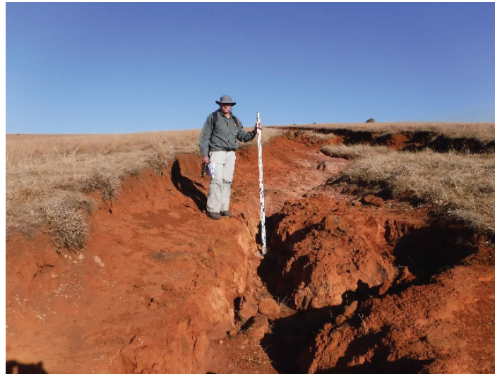
Figure 1 : Donga erosion at an offset site requiring rehabilitation.
