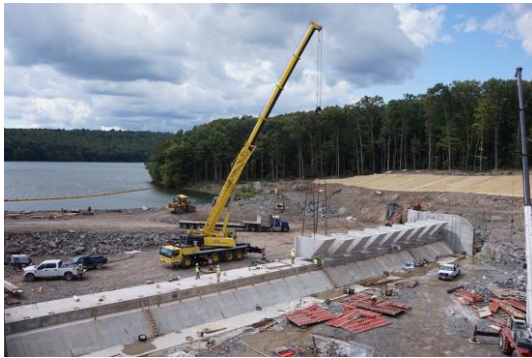
Fig. 14 Fusegate Installation at Pikes Creek F..
