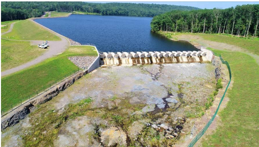
Fig. 16 Completed Auxiliary Spillway at Pikes Creek F..
