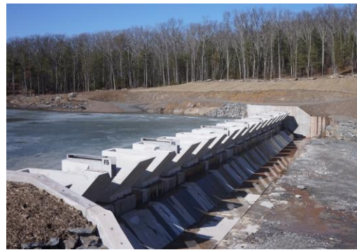
Fig. 15 Completed Fusegate System at Pikes Creek F..
