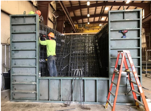
Fig. 11 Custom-made formwork and steel placement F..
