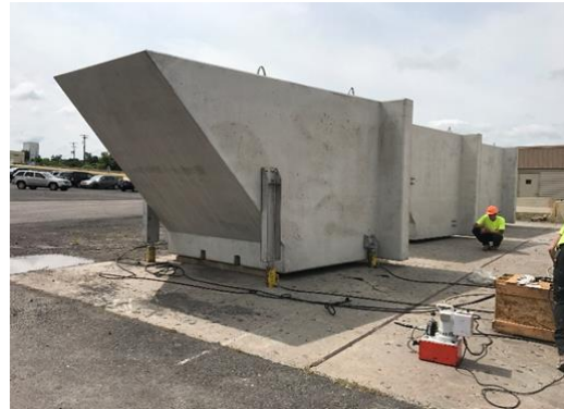
Fig. 12 Fusegate jacking to verify ballast requirements F..
