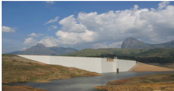
Figure 4 : Kadampara dam after installation of the geomembrane system
