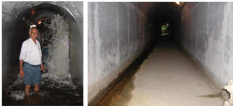
Figure 3 : Drainage gallery before and after geomembrane installation.
