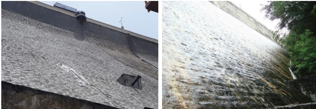
Figure 6 : Downstream side before and after geomembrane installation.
