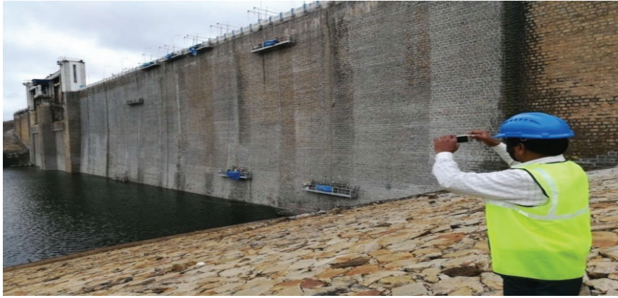
Figure 4 : Upstream face of Sholayar
