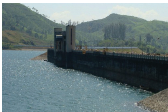
Figure 2 : A view of Sholayar Dam – U/s face
