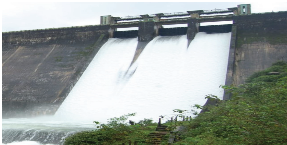
Figure 3 : Spillway portion of Sholayar dam with three gates
