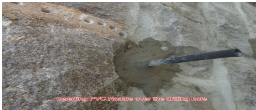
Figure 7 : Injection grouting
