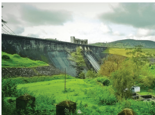
Figure 1 : A view of Sholayar Dam - D/s face
