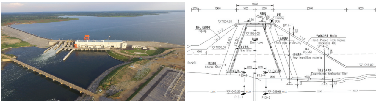
Figure 1 : An aerial view of Isimba Hydro Power Plant; Cross section view of Embankment Dam with installed instruments
