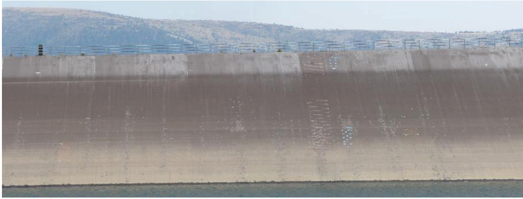
Figure 7 : Arrangement of blisters in clusters extending down the slope.
