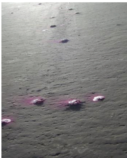
Figure 6 : Blisters developed 4 years after the repairs were carried out
