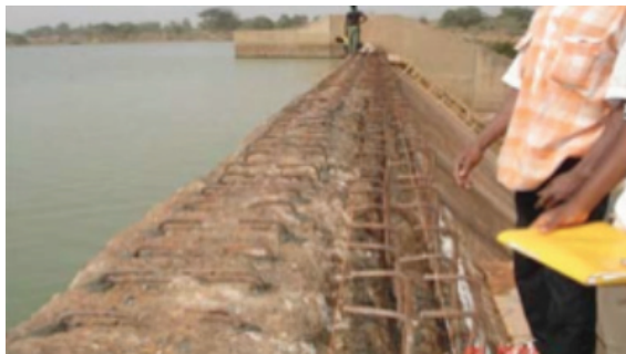
Figure 6 : View of the spillway crest widening operation
