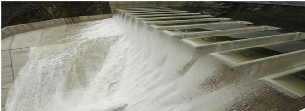
Figure 1 : Piano Key Weir in operation (Laugier, 2016)
