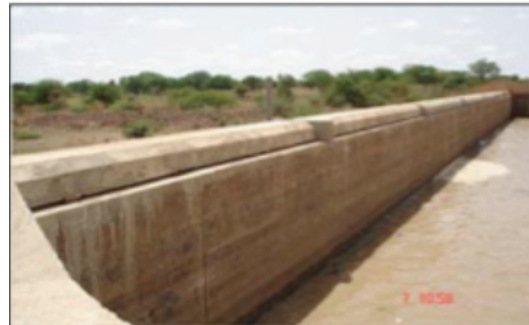
Figure 7 : View of spillway heightened by fuse plugs
