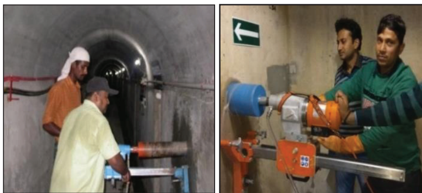
Figure 1 : Concrete Core Extraction in Gallery of Dam
