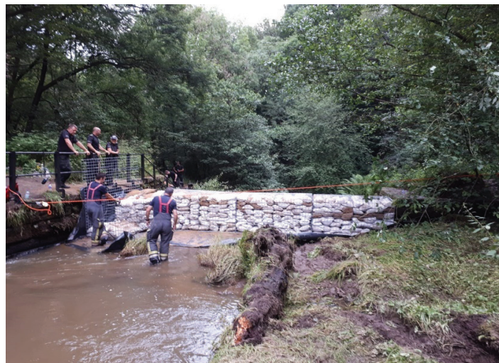
Figure 5 : Inlet weir modifications
