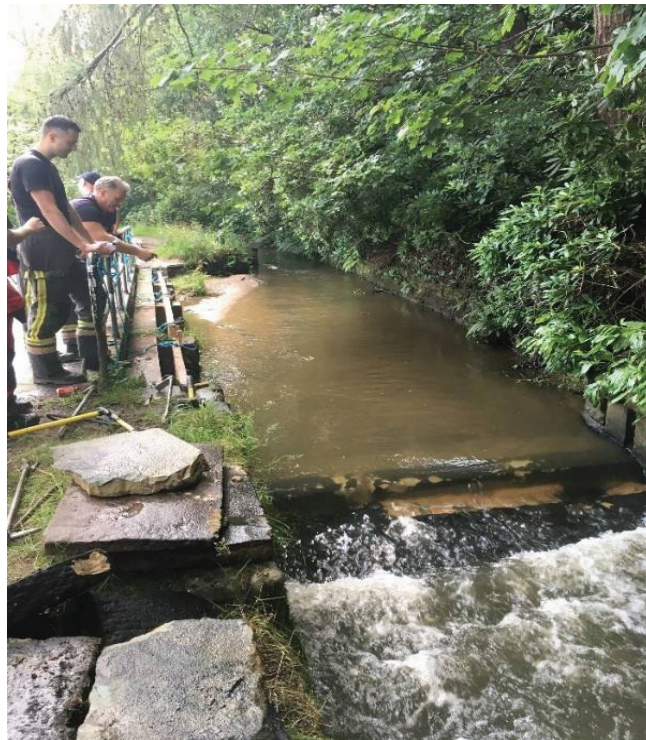
Figure 3 : Bywash side weir
