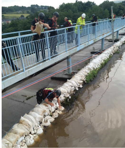
Figure 4 : Photo of sandbagging the auxiliary weir crest
