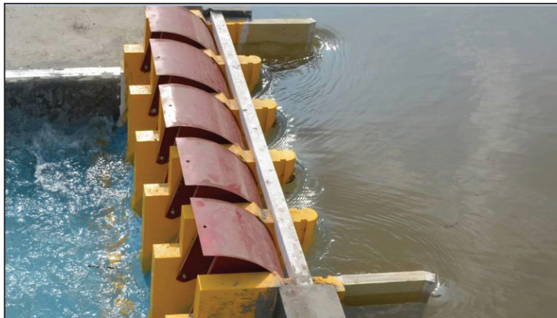
Photo 9 : Approach flow condition of existing left spillway of main dam
