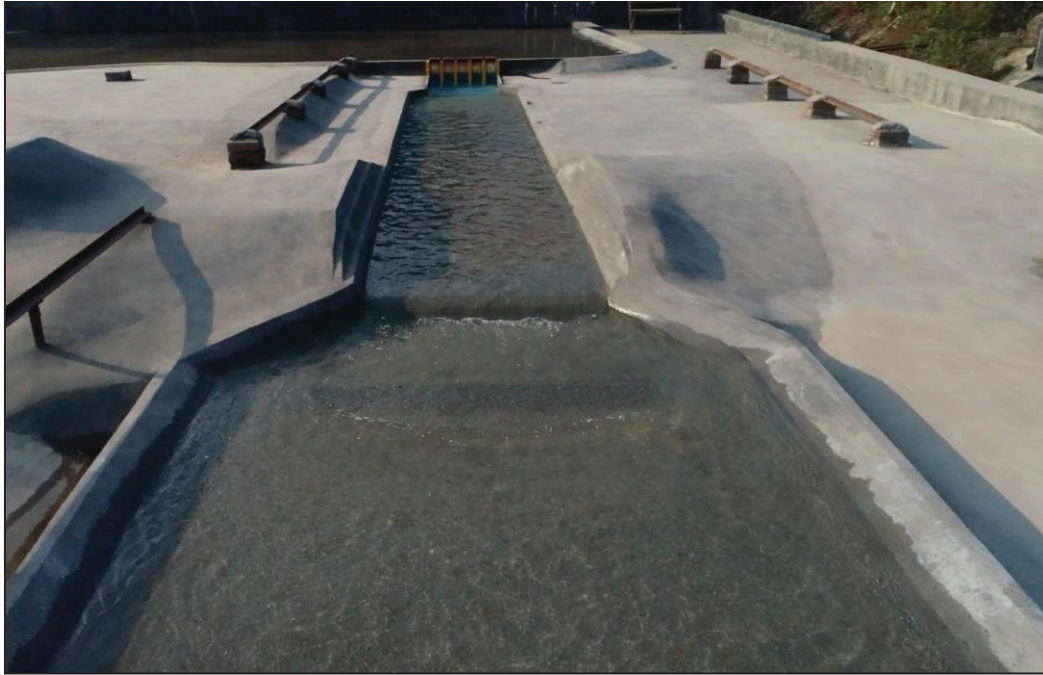
Photo 13 : Flow condition in the entire spill channel
