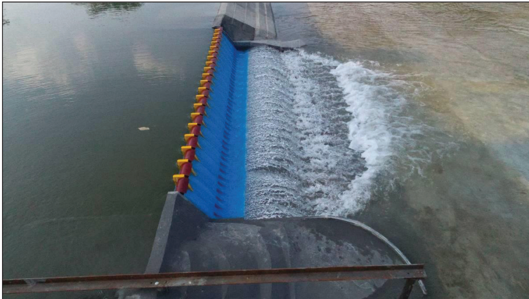
Photo 14 : Flow condition in the spill channel from RD 857 m to RD 936.26 m
