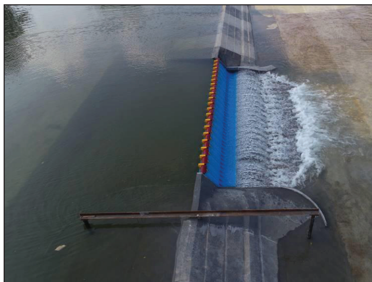
Photo 10 : Upstream flow condition near the left and right training wall
