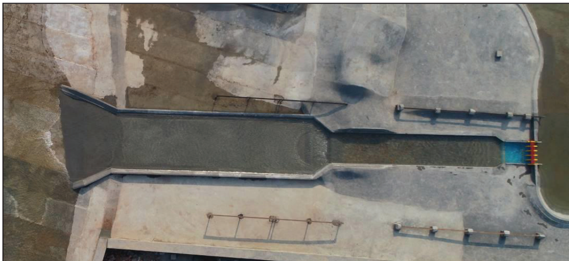
Photo 12 : Performance of Stilling basin of additional spillway
