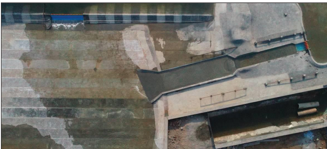
Photo 15 : Performance Ski-jump Bucket of existing left spillway of main dam
