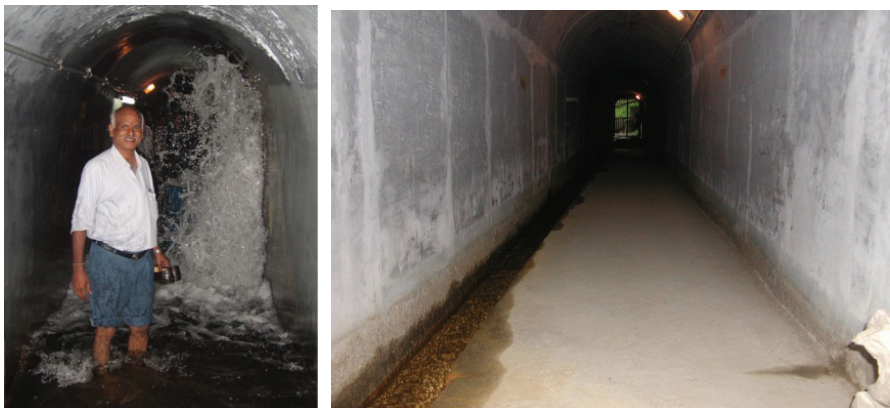
Figure 3 : Drainage gallery before and after geomembrane installation.
