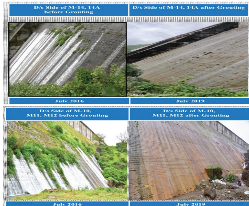
Picture 1 : Leakage Comparison before and after repair work.
