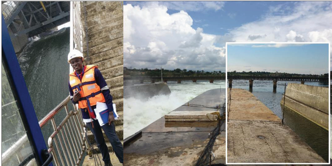
Figure 9 : Showing the right opening at 70% opening with the corresponding downstream water level rise
