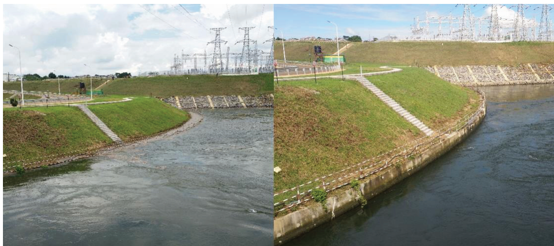
Figure 10 : Showing the downstream water levels during the test and after reinstatement process
