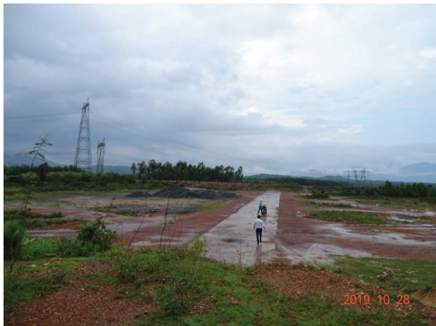
Figure 7.1 : Newly constructed emergency spillway at Phu Vinh Dam
